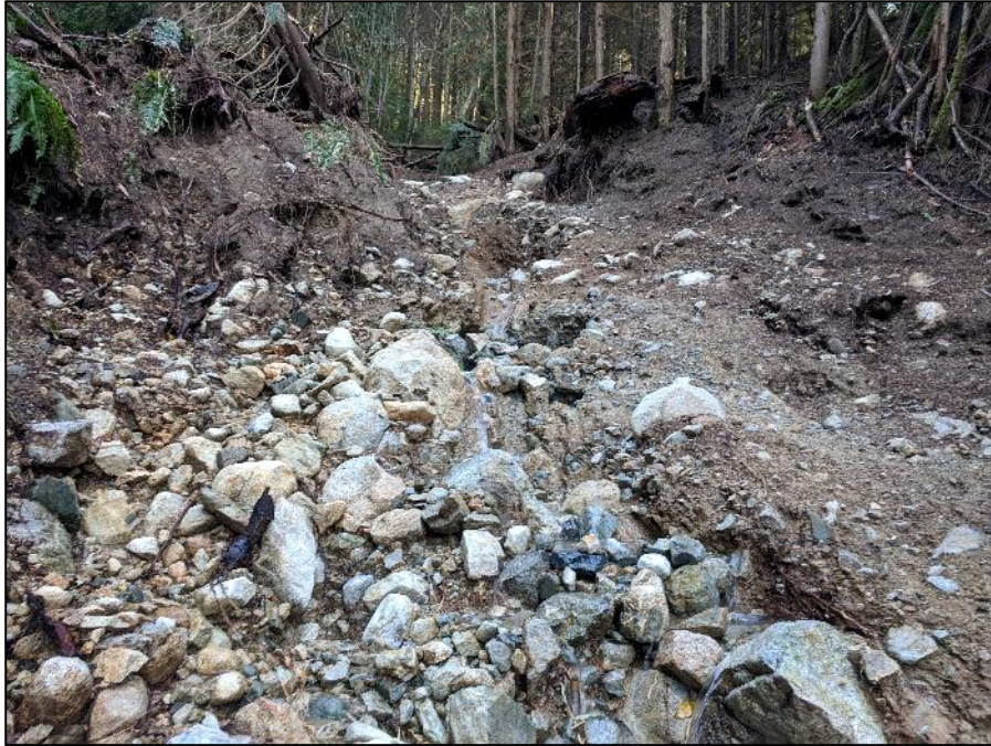
Photo 4: Looking up the landslide path. The slide scoured through the compacted or cemented till. The slope gradient is about 50%. The path is about 5 m wide.
