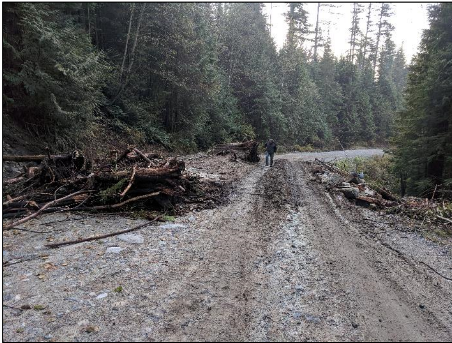
Photo 15: Looking down the Lost Creek FSR near where the landslide crossed the road. The slide entered the road on the left and deposited large woody debris and fine textured sediment on the road, but did not completely block the road.
