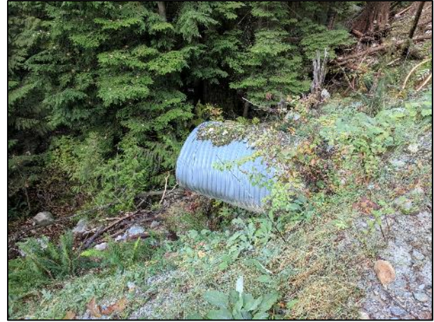
Photos 13 and 14: The culvert near where the slide crossed Lost Creek FSR. Photo 13 shows the lower culvert, with water flowing in the pipe. Photo 14 shows the upper culvert that has a blocked inlet, with no water flowing through the pipe.
