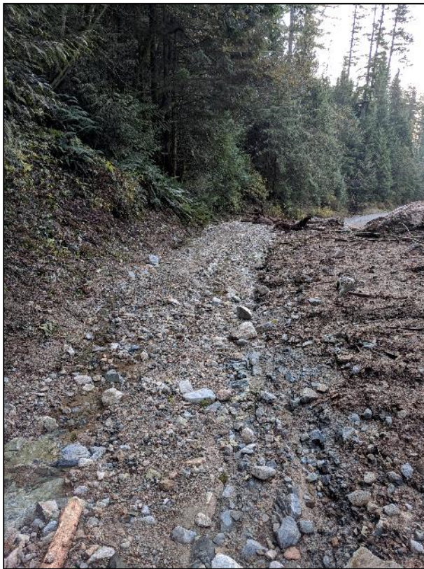
Photos 17 and 18: Landslide debris filled in the ditch between where the slide hit the road and the upper culvert. Between the upper and lower culverts, there was less sediment in the ditch.
