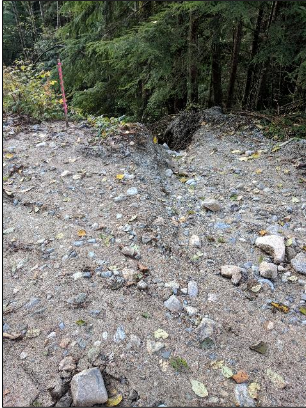
Photos 10 and 11: The culvert outlet, about 70 m from the slide crossing and the washout.
