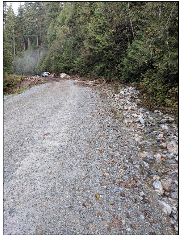
Photos 17 and 18: Landslide debris filled in the ditch between where the slide hit the road and the upper culvert. Between the upper and lower culverts, there was less sediment in the ditch.
