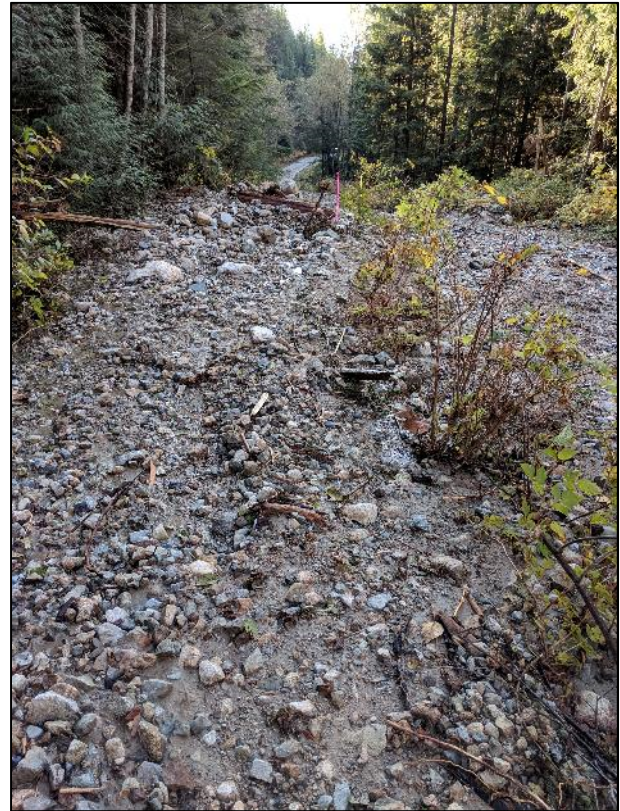
Photos 8 and 9: The slide path reaching Lost Murdo FSR. Some of the slide debris flowed down the road and some crossed the road.
