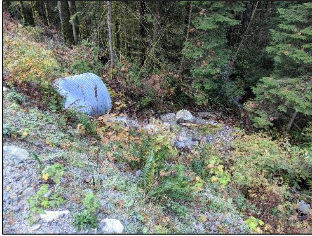
Photos 13 and 14: The culvert near where the slide crossed Lost Creek FSR. Photo 13 shows the lower culvert, with water flowing in the pipe. Photo 14 shows the upper culvert that has a blocked inlet, with no water flowing through the pipe.
