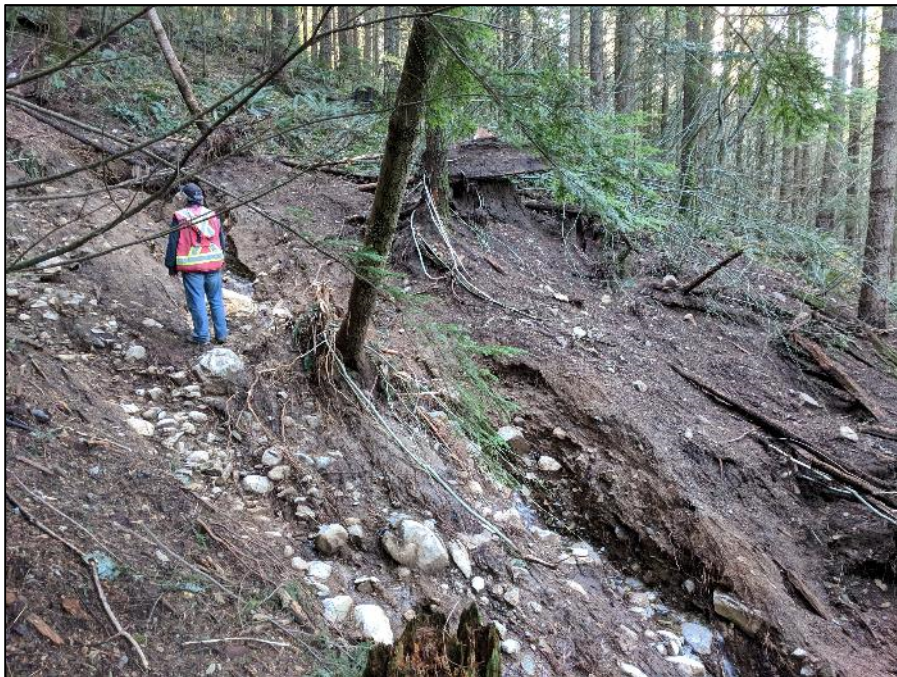
Photo 5: A wide part of the landslide track, with organic material and fine sediment depositing in the forest at the edge of the main path. The slide incised about 1 m. Slope gradients are about 40%.
