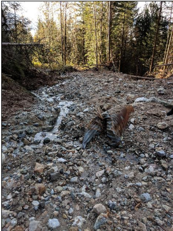
Photos 6 and 7: Crushed pipe inlet where at the Lost Murdo FSR. Water is flowing down the road instead of across it. The end of the crushed CMP, where part of the slide continued down the stream channel to The Lost Creek FSR.
