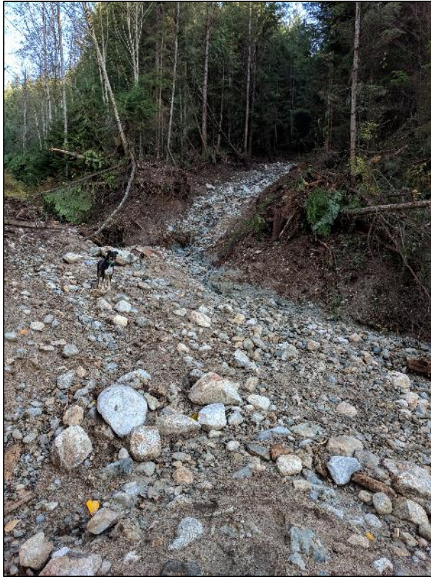
Photos 8 and 9: The slide path reaching Lost Murdo FSR. Some of the slide debris flowed down the road and some crossed the road.
