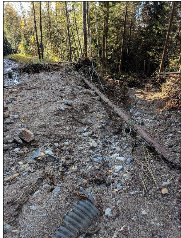
Photos 6 and 7: Crushed pipe inlet where at the Lost Murdo FSR. Water is flowing down the road instead of across it. The end of the crushed CMP, where part of the slide continued down the stream channel to The Lost Creek FSR.
